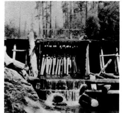
Figure 31.—A splash dam at Austin Place, Hamilton Creek, Oregon, August 16, 1907. Such dams were used to regulate the flow of water to float logs down a stream to the mill. (Historical photo, courtesy of the Horner Museum, Oregon State University.)
