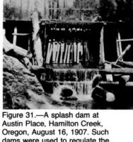
Figure 31.—A splash dam at Austin Place, Hamilton Creek, Oregon, August 16, 1907. Such dams were used to regulate the flow of water to float logs down a stream to the mill. (Historical photo, courtesy of the Horner Museum, Oregon State University.)
